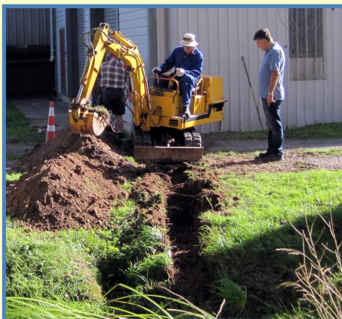
Above: The 'small yellow digger' on 14 th May, digging the trench for a second storm water outlet from the workshop.
